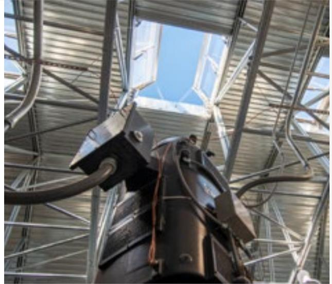
**Pictured:** The wide opening of the BILCO roof hatches made it easy for the facility to install large pumps and the hatches provide convenient access for future pump replacement.
